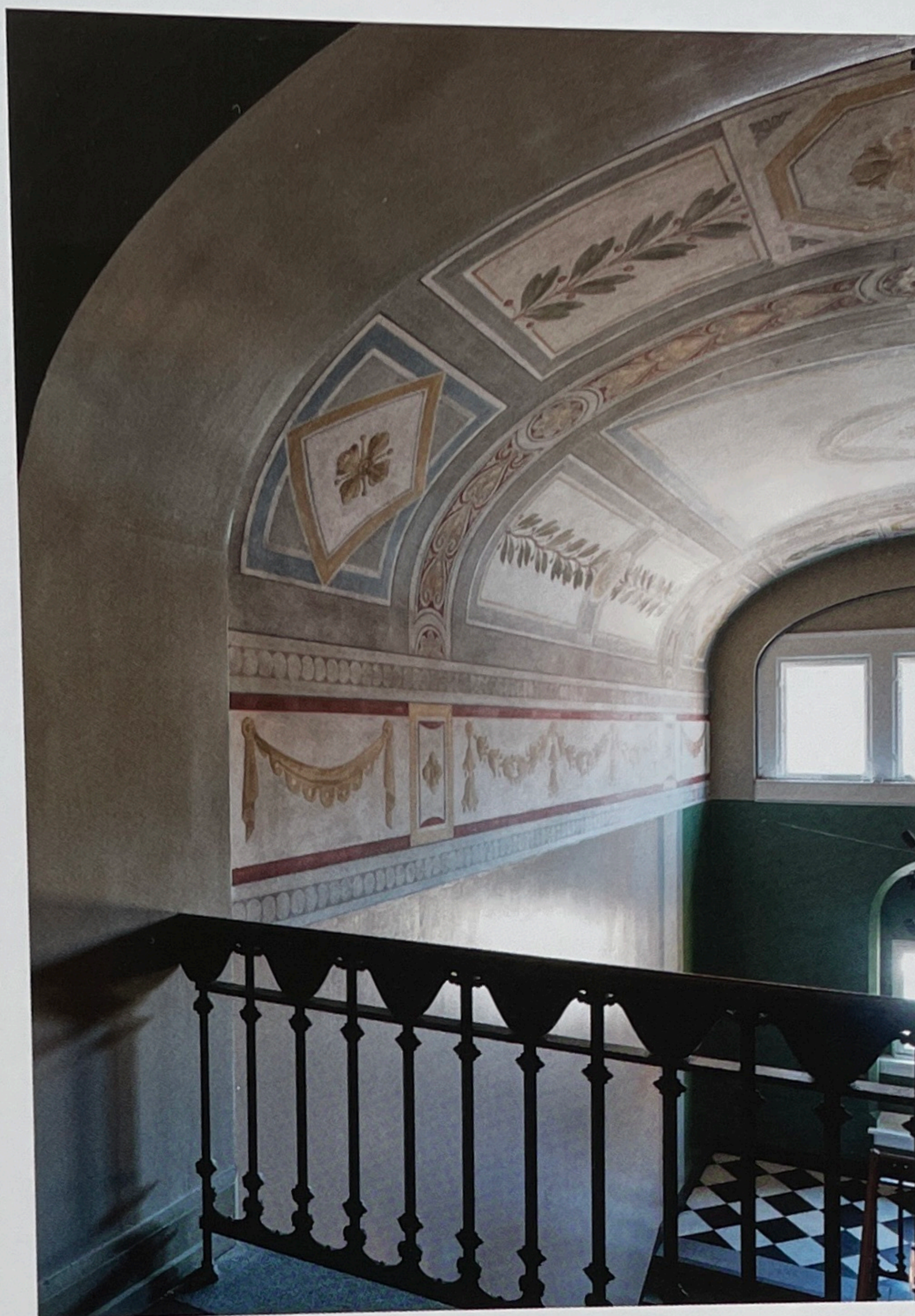
Detail of the ceiling motif repeated throughout the house. The decoration is meant to create the illusion of murals from Italian Renaissance palaces in secco and fresco techniques.
